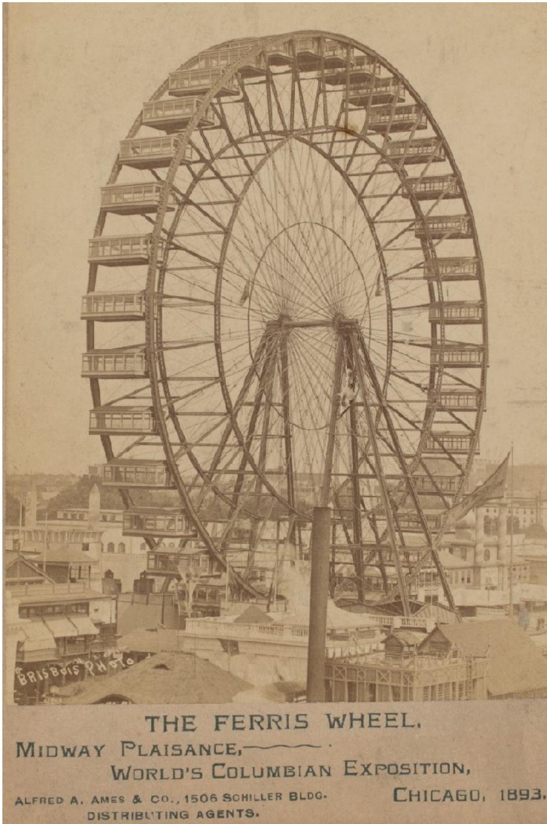
The Ferris wheel was invented in 1893 by George Washington Gale Ferris. He was an engineer and bridge builder. This Ferris wheel was 264 feet tall and had 60 cars. Each car was the size of a school bus and could carry 60 passengers. IChi-73008
