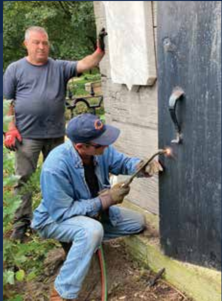
Top: Openlands volunteers joined by US Congressman Mike Quigley plant trees at the Richard M. and Shirley H. Jaffee History Trail. Photograph by Terrance Lewis, October 28, 2023. Bottom: Chicago Park District metal workers repair a steel door on the Ira Couch tomb. Photograph by Eric Miller, October 5, 2023.
