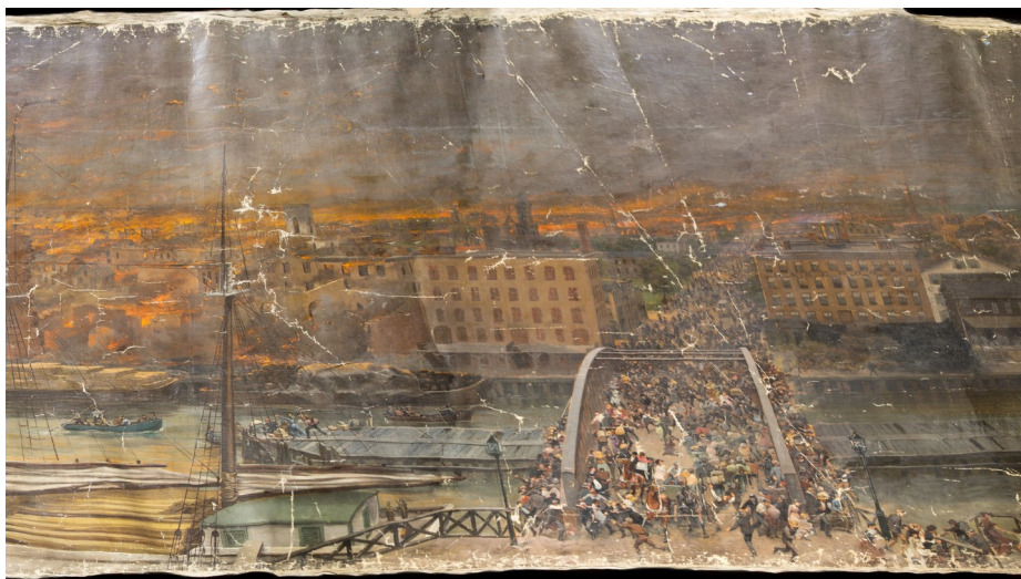
Cyclorama Section — Rush Street Bridge
