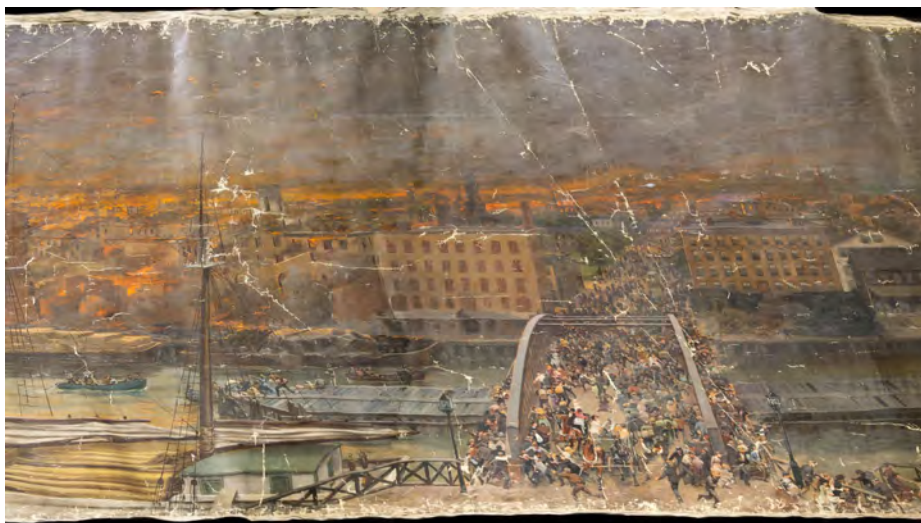
Cyclorama Section — Rush Street Bridge
