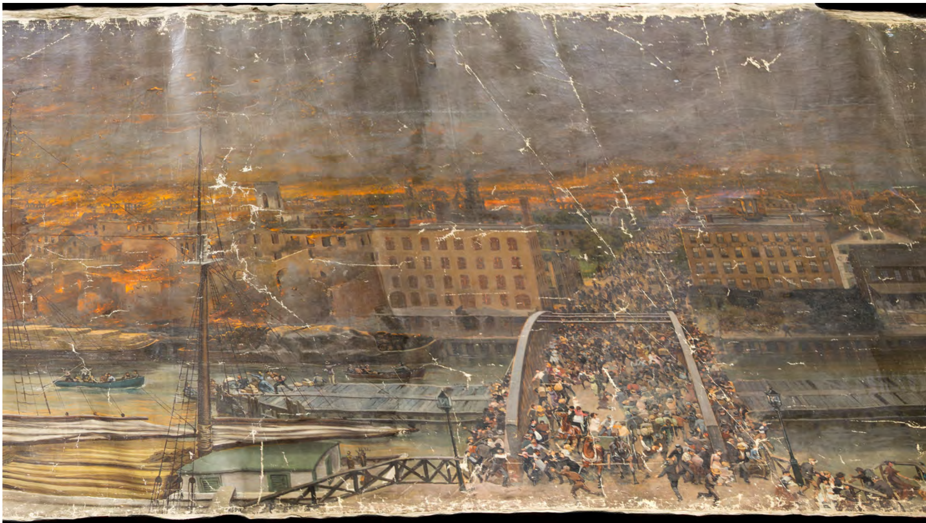
Scene at the Rush Street Bridge, Cyclorama of the Great Chicago Fire , 1871.
